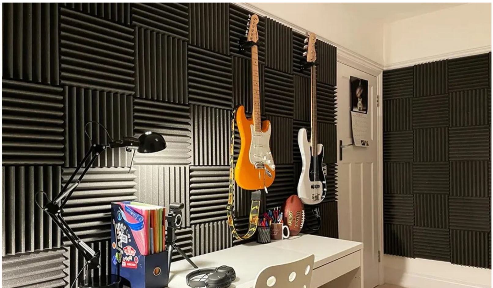
An example of how FOAM panels are used to treat a room.
